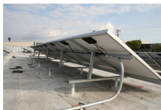
Figure 15: Penetrated System, high tilt example. typ 3 - 4 lbs/sq.ft. Courtesy of Mangan.
