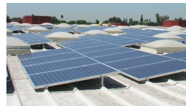
Figure 16: Clamped System, standing seam metal roof. typ 3 lbs/sq.ft. Courtesy of Mangan
