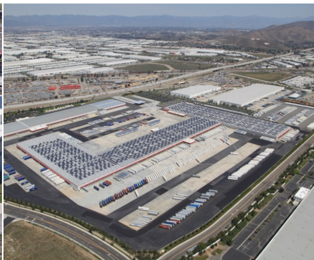
Figure 2: 3MW AC in Mira Loma, California, USA. Courtesy of Mangan Renewables
