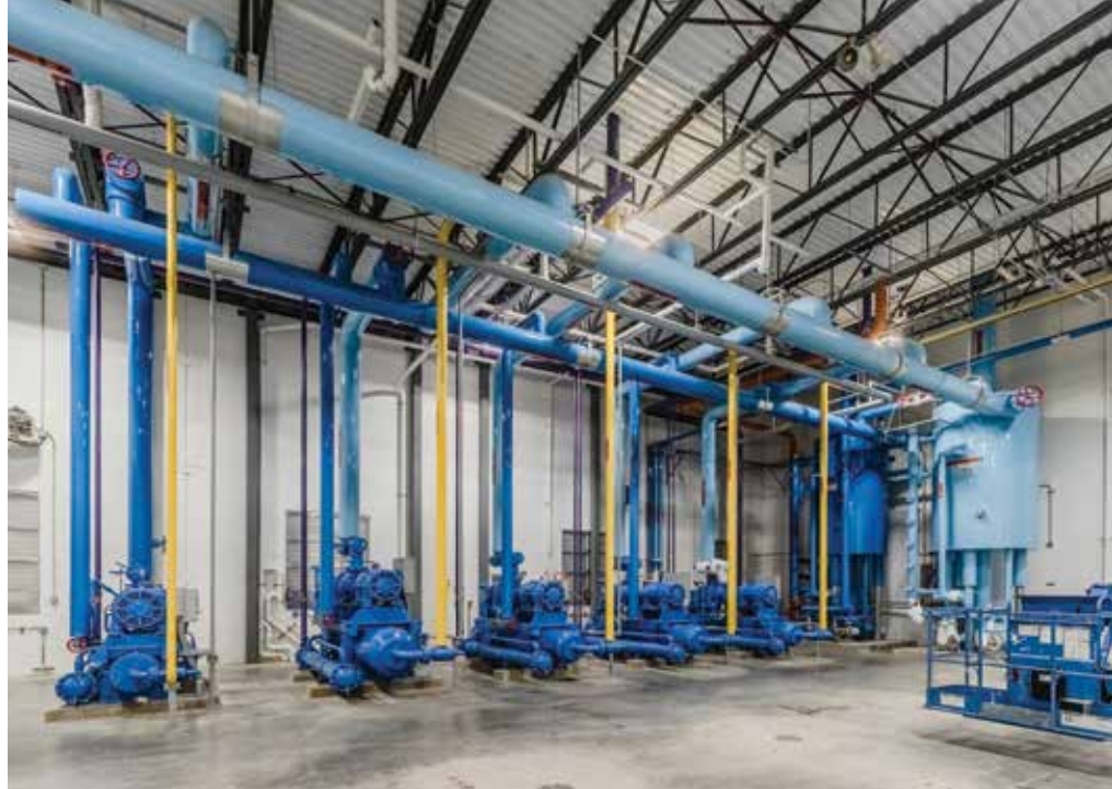
The plumbing and electrical in the engine room was encased in flowable grout instead of concrete to save time. (Photo courtesy of Primus Builders, Inc.)
