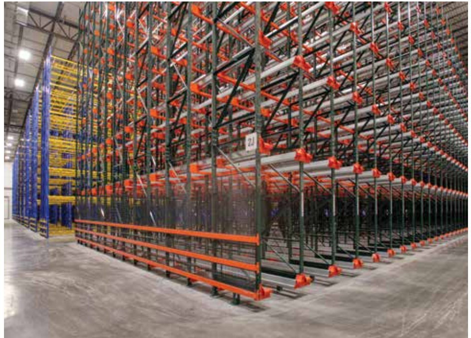
At 51-feet high, the 312,000-square-foot building was designed to offer Americold maximum flexibility in its cold storage options. (Photo courtesy of Primus Builders.)
