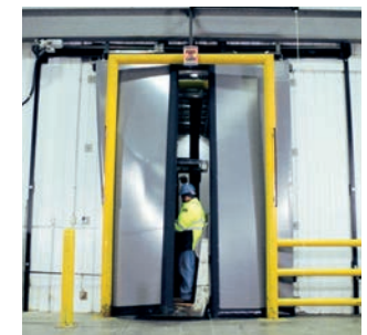
Flexible, impactable insulated panels ( k= 0.568 \text{ W/m}^2\text{K} )
