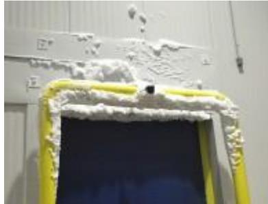
**Picture 03. Frost Due to Condensation Problems**
