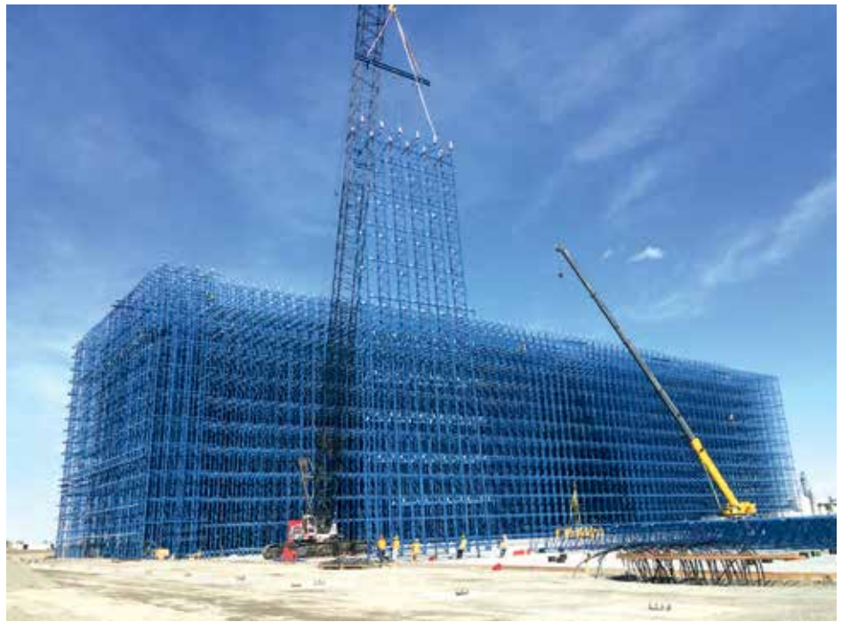
Preferred Freezer’s Richland, Washington facility’s 116-foot-tall building with over 117,000 total pallet storage positions is the largest public refrigerated warehouse in North America.
