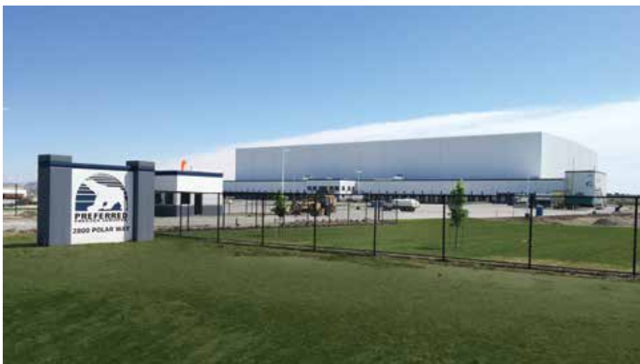
The decision to install a low-oxygen fire protection system for Preferred Freezer’s automated freezer facility in Richland, Washington was based on cost-effectiveness and need to ensure the facility remained operational 24/7.
