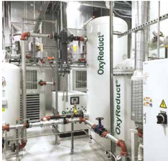
Left: By generating nitrogen from the ambient air onsite, the OxyReduce® system minimizes space needed for low-oxygen fire prevention and makes it possible to relocate the system if space is used for a different purpose. Right: Low-oxygen fire protection is ideal for storage racks at or over 75 feet – a height that is difficult to protect with traditional systems.
