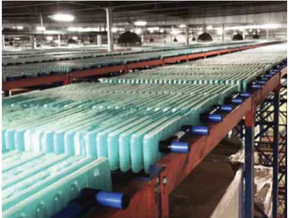
The Thermal Energy Storage technology installed at Dreisbach Enterprises in Richmond, California. (Photo courtesy of Viking Cold Solutions.)
