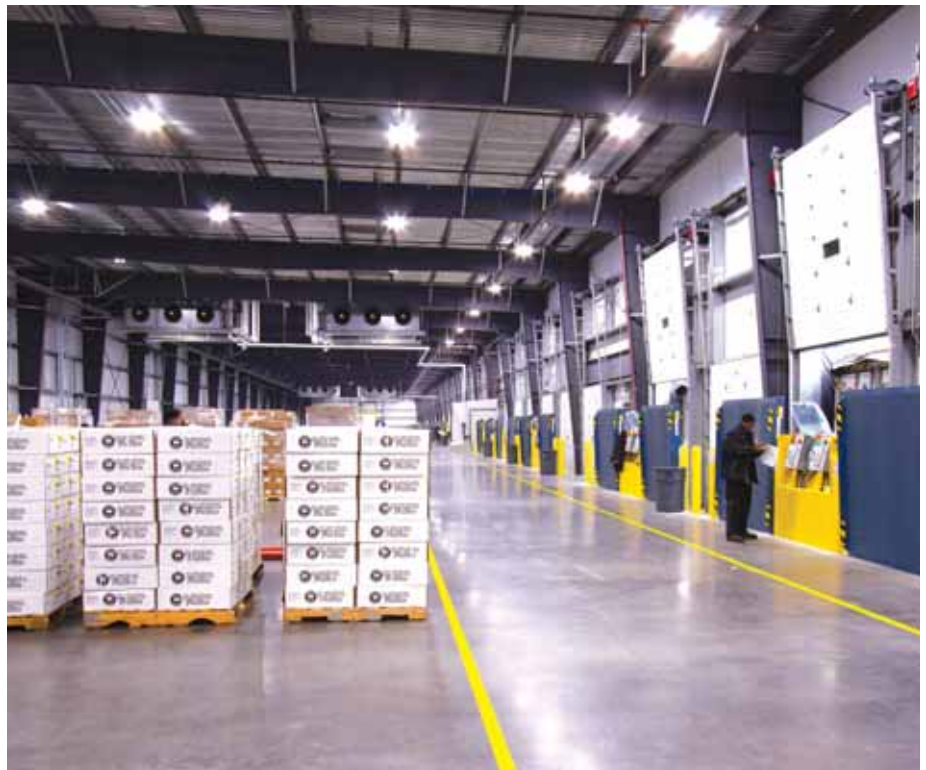
Two thirds of the entire facility is comprised of a winged refrigerated loading dock, allowing for product transloading in optimal conditions. (Photo courtesy of Fisher Construction Group.)
