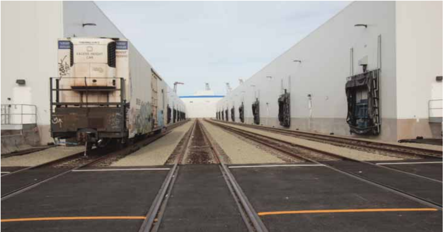
One hundred and eight rail and truck doors in the refrigerated cross-dock were designed with a complex set of interlocks to help maintain the cold chain. (Photo courtesy of Fisher Construction Group.)
