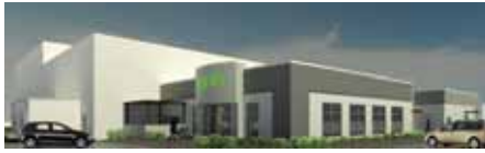
GAB Operations, constructed by A M King in south Texas, United States. (Photo courtesy of A M King.)
