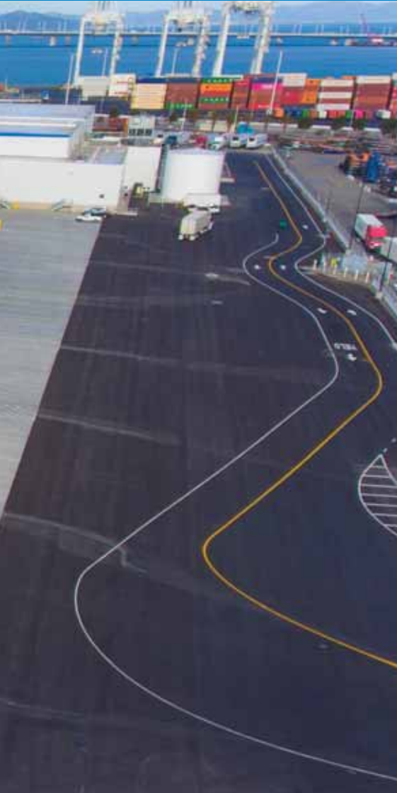
Port of Oakland, California, United States. (Photo courtesy of Fisher Construction Group.)
