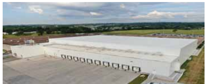
Winchester Cold Storage, Winchester, Virginia
