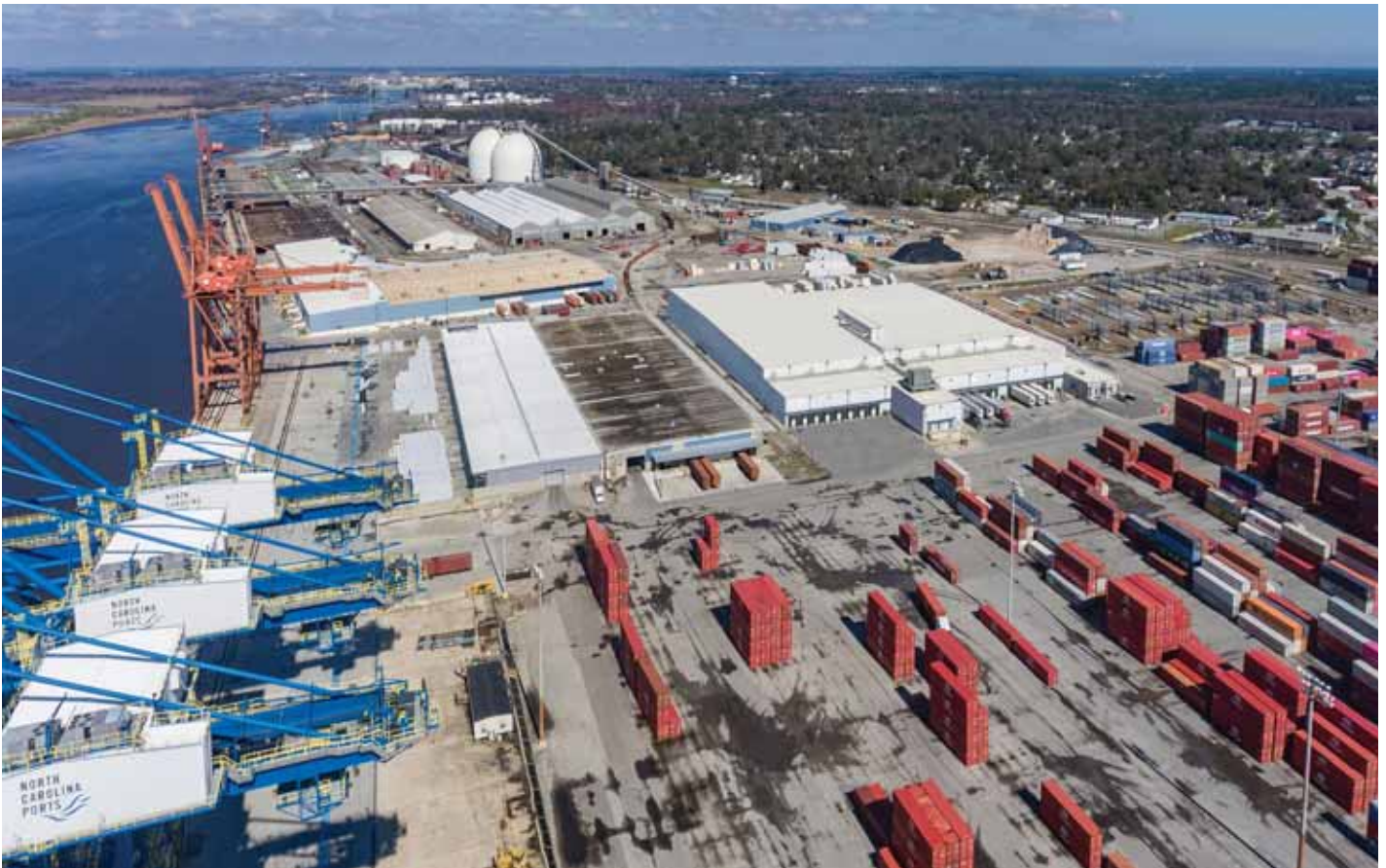
Port of Wilmington, North Carolina, United States. (Photo courtesy of Port of Wilmington Cold Storage.)
