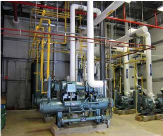
We have an Ammonia/ $\text{CO}_2$  system installed in the Winchester Cold Storage facility in Winchester, VA.
