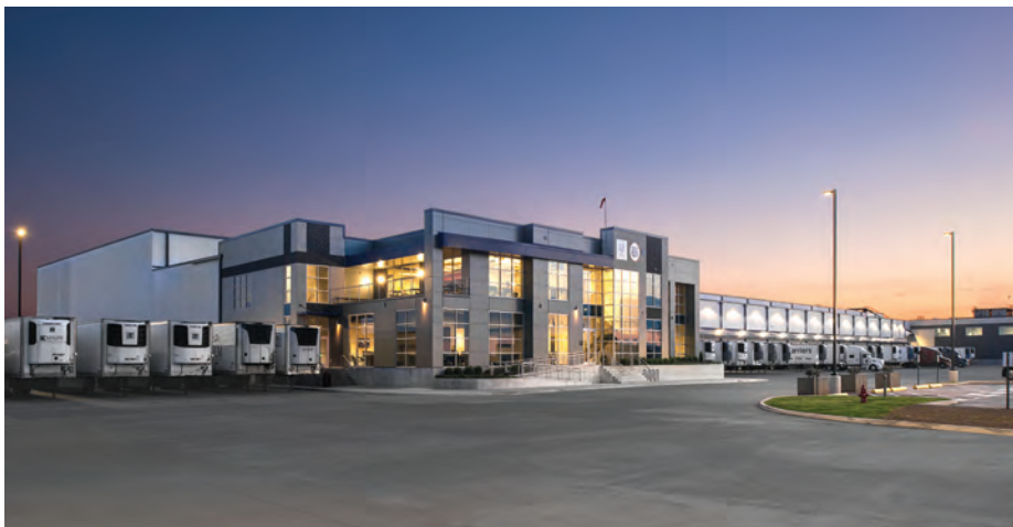
Primus installed solar-reflective materials to the U.S. Cold Storage facility in Covington, Tennessee, to ensure the building’s roof and paved areas do not create an irregular “heat island” in a rural setting. Light pollution was mitigated with outdoor fixtures that cast light downward and not beyond 15 feet of the property. (Photo courtesy of Primus Builders.)
