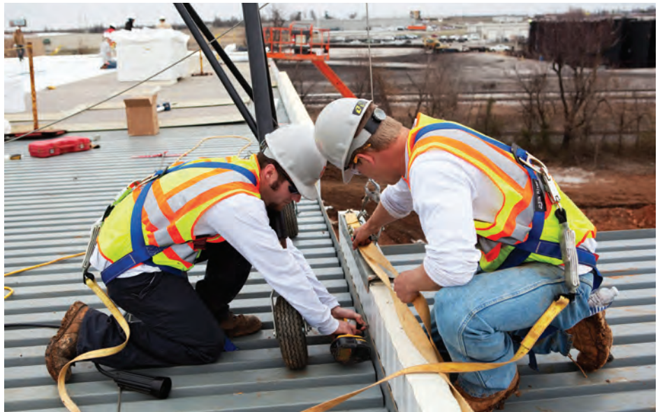
Recording and analyzing near-misses is essential in determining whether hazard controls are adequate.
