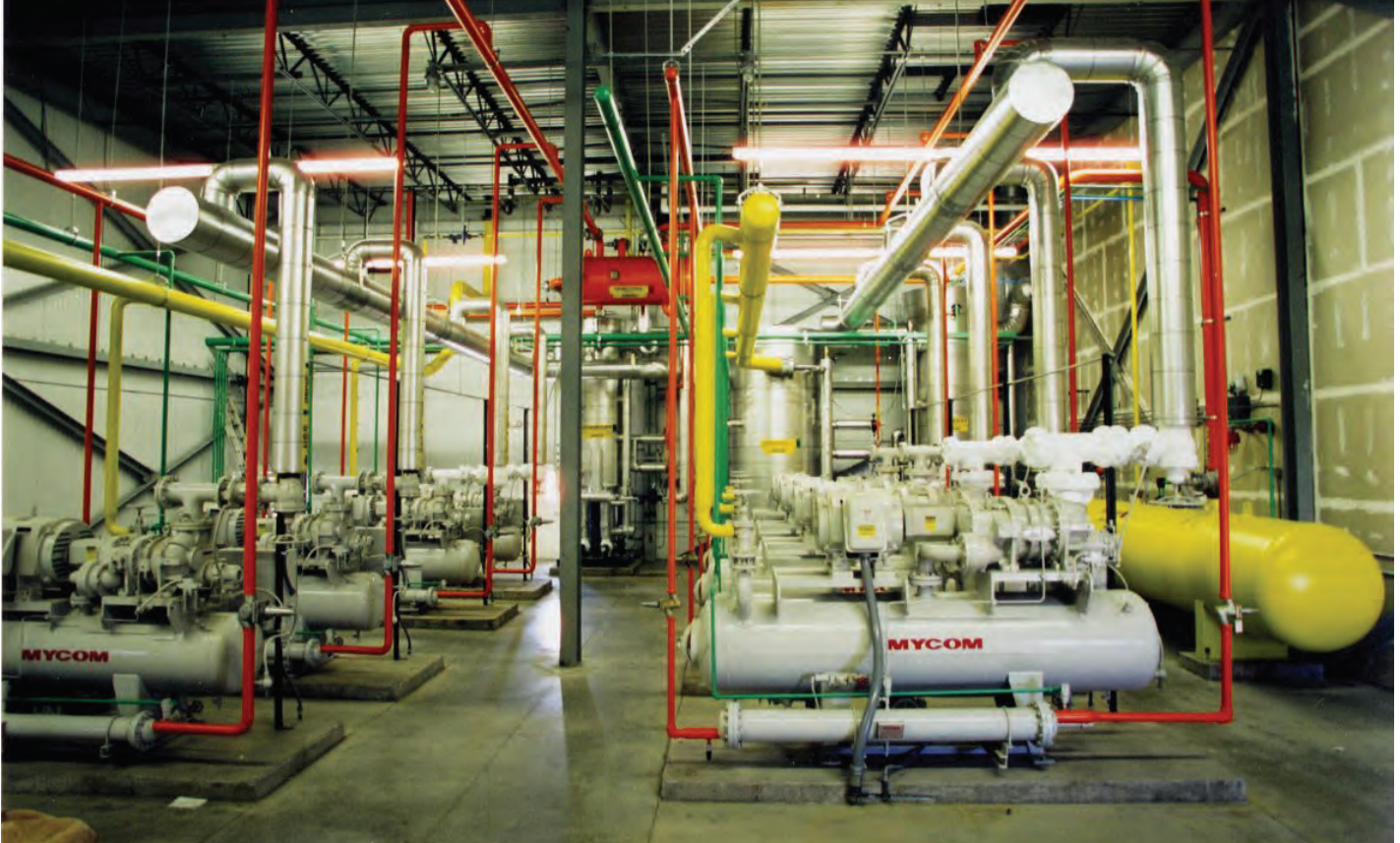
Refrigeration equipment is one of the key energy-consumption areas addressed in a new guidance document the IACSC-IARW Construction/Codes Committee submitted to the U.S. Green Building Council to help the group create LEED certification standards for refrigerated warehouses.
