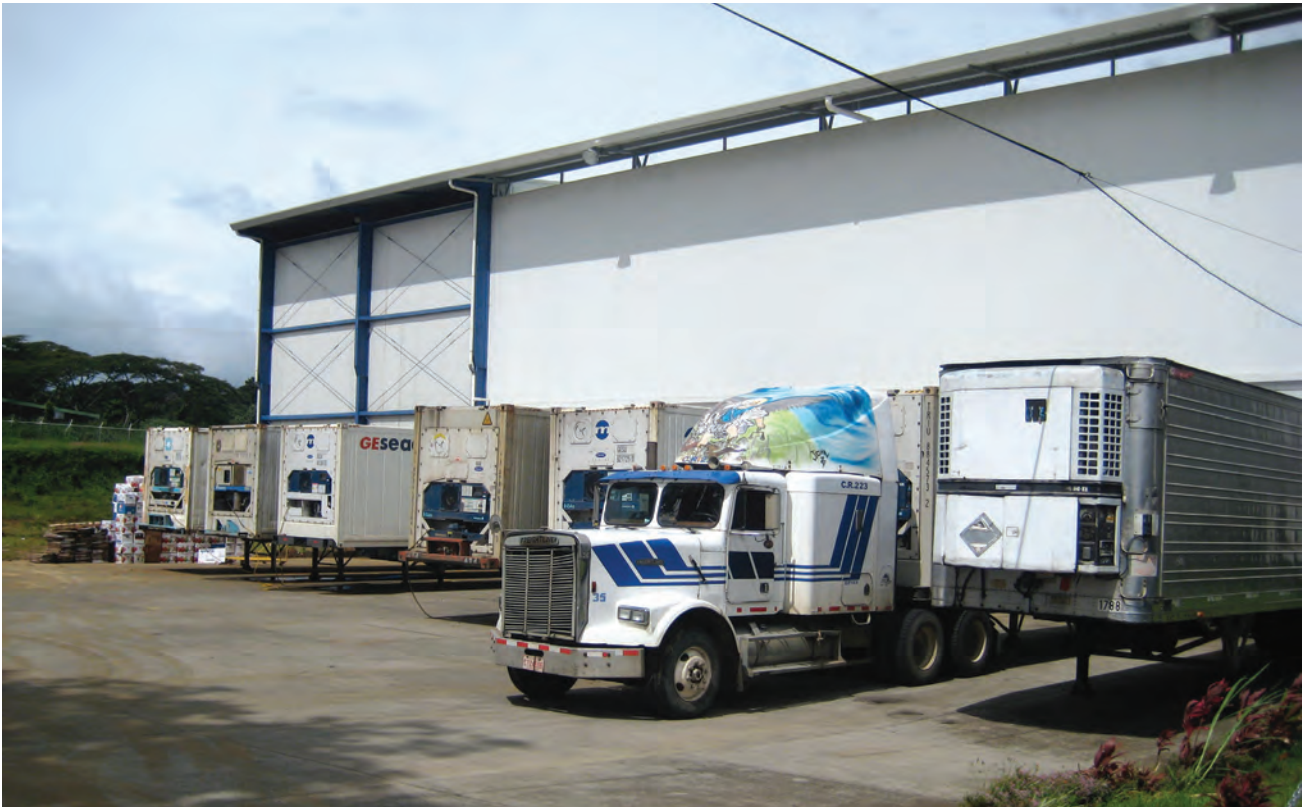
The loading dock at Polo Norte Cold Storage, Costa Rica. Over 500 trucks ship in fresh apples from Chile for the Christmas holiday season. The majority of the trucks arrive with gen-sets as the delays at the ports can be long. (Photo courtesy of Mark Washburn.)
