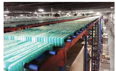
TES cells filled with phase change material installed on top of the racks in Dreisbach's freezer. (Photo courtesy of Viking Cold.)
