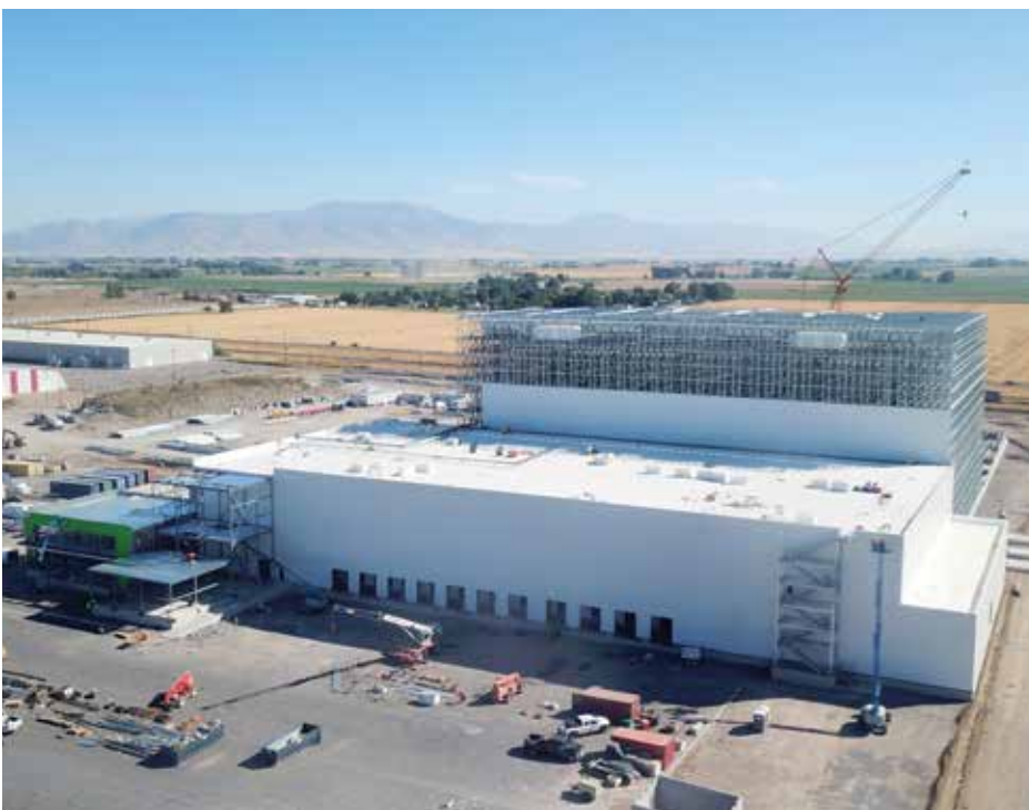
Left: The second fully automated high bay cold facility in the States is under construction in Idaho. Right: The facilities rely on automated storage and retrieval systems to move and store product in the high-bay warehouse. (Photos courtesy of NewCold.)
