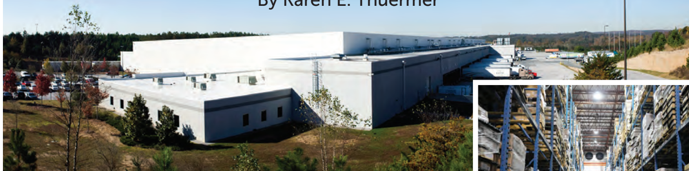
Americold's warehouses are an integral part of the supply chain connecting food producers, processors, distributors, and retailers to the end consumer. (Photo courtesy of Americold.)
