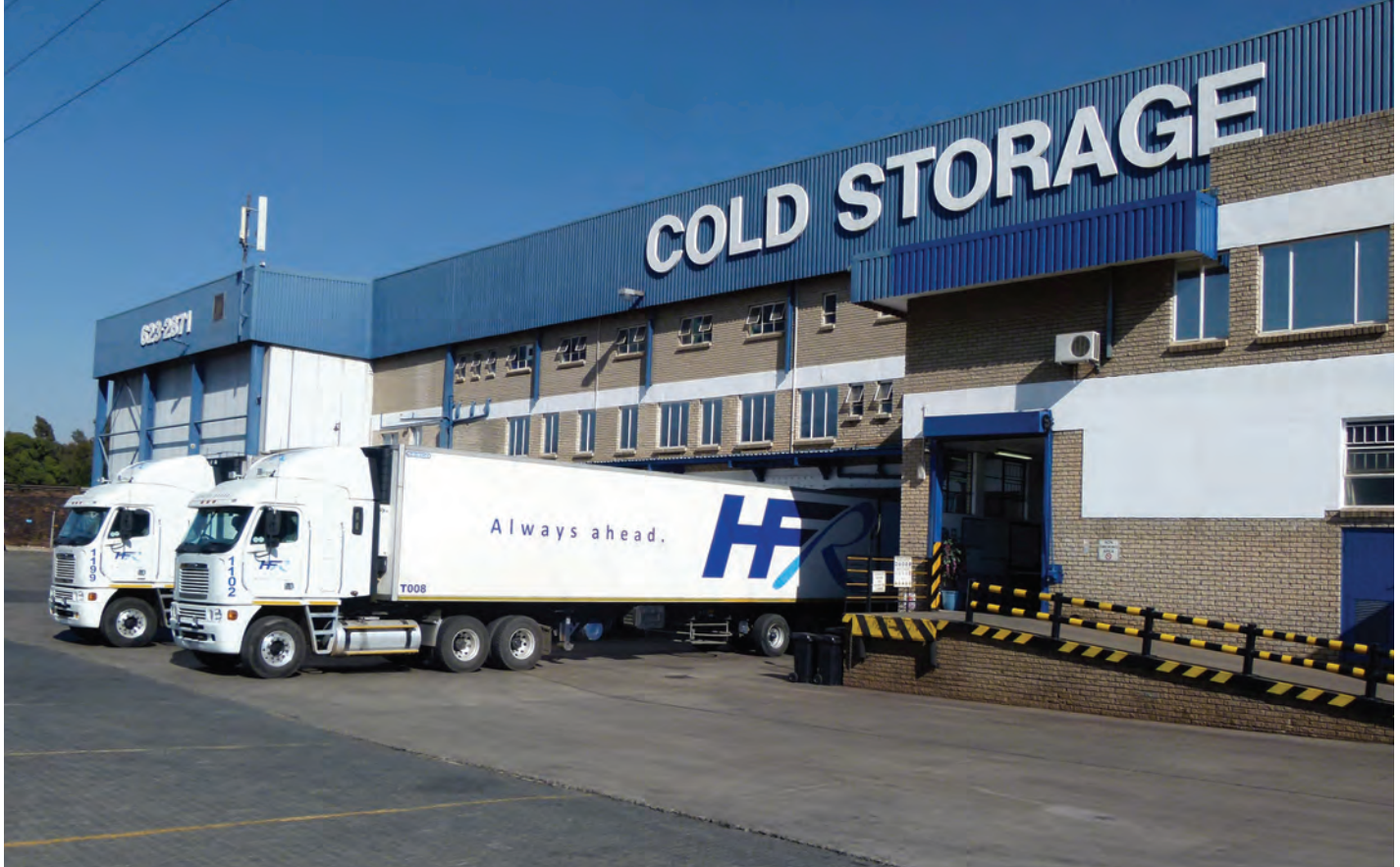
A large public cold storage facility in Johannesburg. (Photo courtesy of SARDA.)
