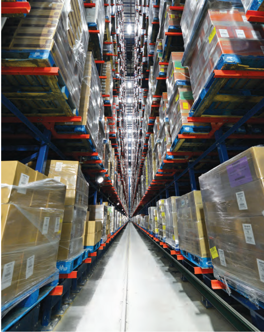
Conestoga Cold Storage's fully automated Mississauga facility stands 120-feet tall with three AS/RS cranes servicing over 12,000 pallet positions. (Photo courtesy of Conestoga Cold Storage.)
