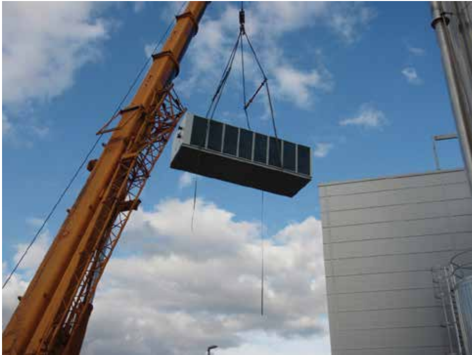
The low-charge, air-cooled Azanefreezer package, shown here being lifted into position onto a building roof, is one of several low-ammonia charge systems examined in a recent GCCA white paper. These condensing units are typically used for freezer warehouse applications.
