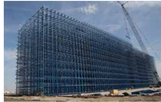
This Preferred Freezer Services cold storage facility will be the largest public refrigerated warehouse in North America.
