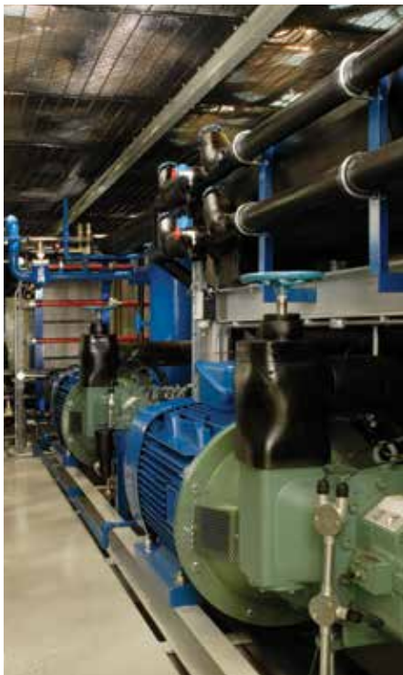
The inside of the low-charge, air-cooled Azanechiller package. These chiller packages are used to chill a secondary fluid for temperature-controlled storage, process cooling or HVAC applications.
