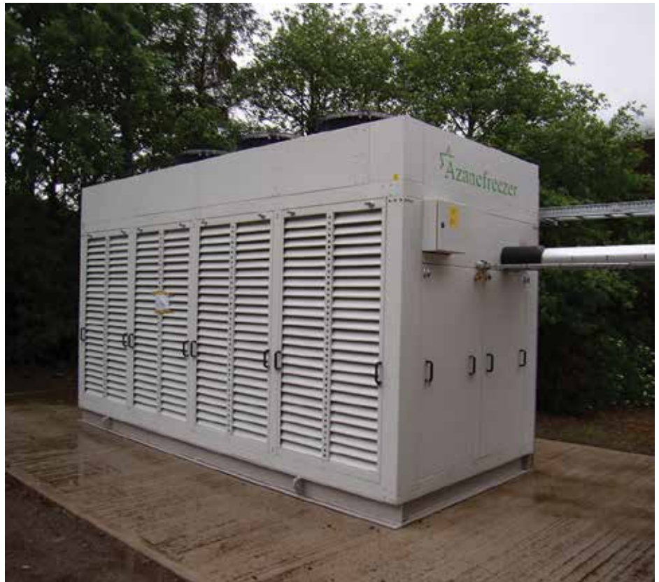
The Azanechiller package installed and ready for use.
