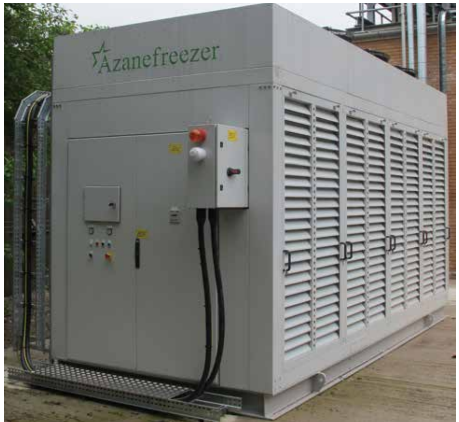
One of the low-charge ammonia packages that are used to replace R-22 refrigeration systems for freezer warehouses.
