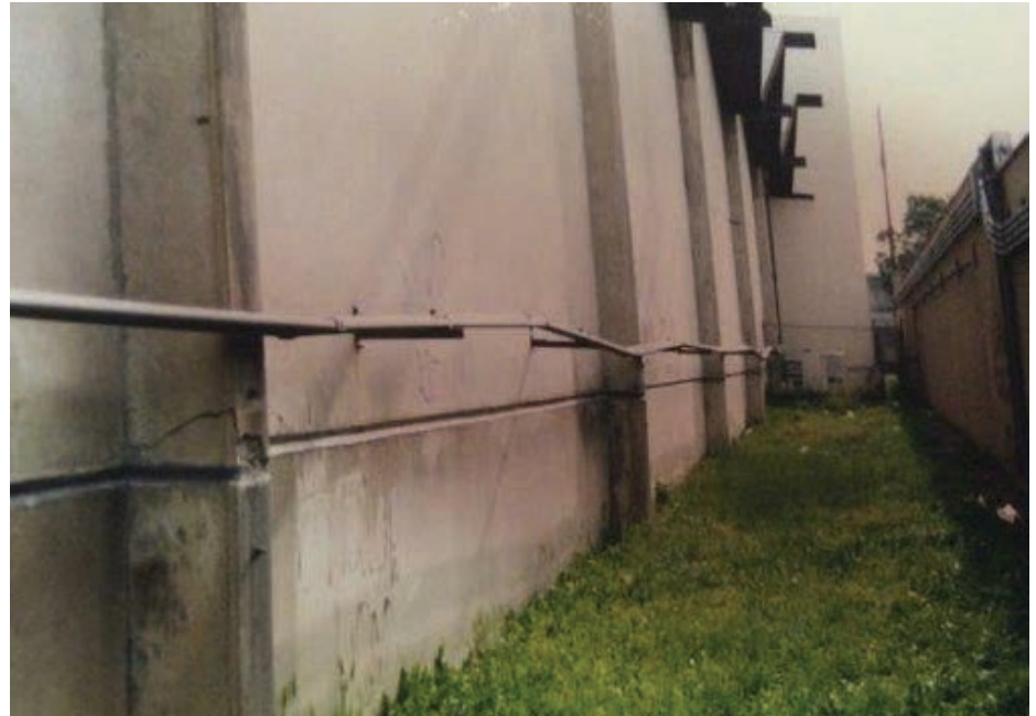
Floor freezing led to this buckled wall and cracked pilaster. (Photo courtesy of Bonar Engineering & Construction Co.)
