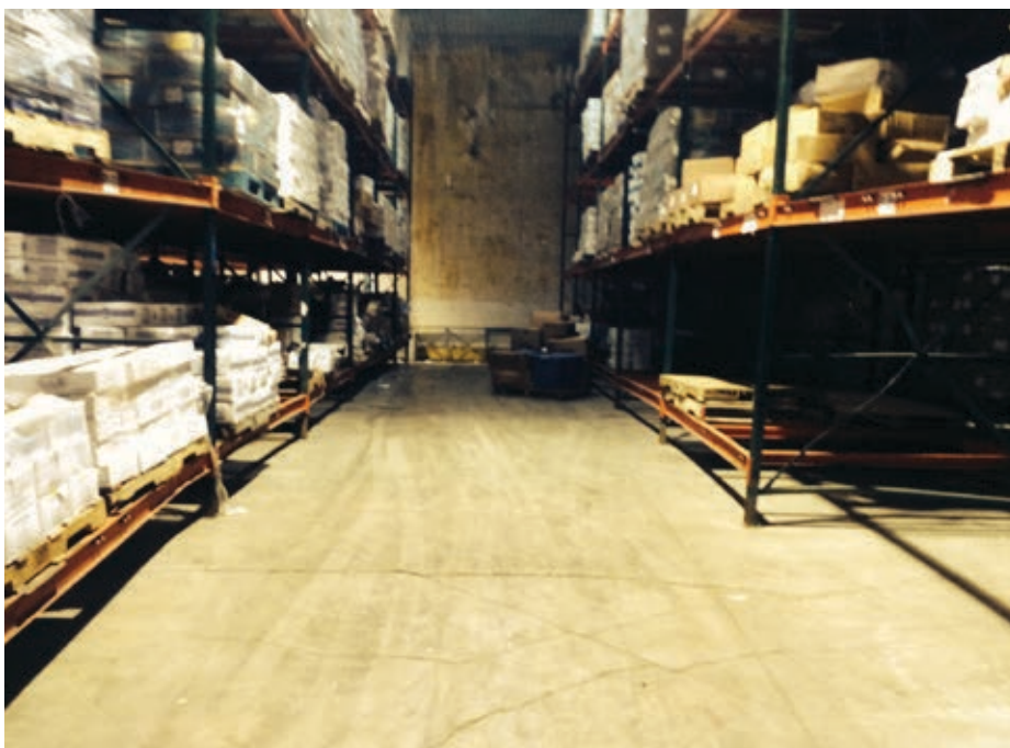
An example of floor heaving in Puerto Rico. (Photo courtesy of Bonar Engineering & Construction Co.)
