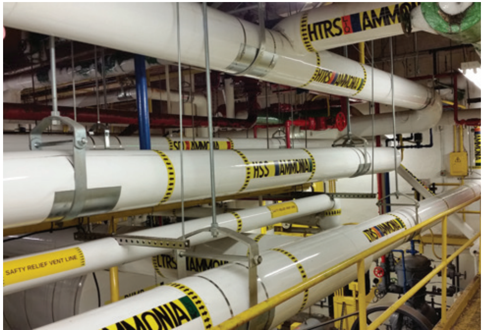
The presence of ammonia used in warehouse refrigeration systems makes it essential that warehouse managers meet with local emergency response officials to review how and where it is used so that any leak in the system can be addressed appropriately. (Photo courtesy of Sodus Cold Storage.)
