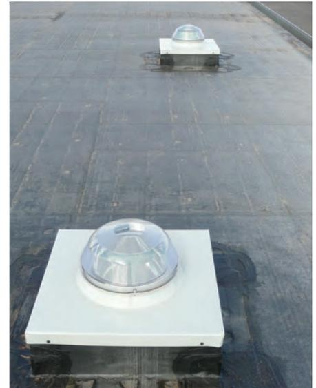
Solar tubes placed on the rooftop collect sunlight and transfer it to fixtures that look like fluorescent lights in office spaces below and are more energy efficient than skylights. (Photo courtesy of ARCO Design/Build Inc.)
