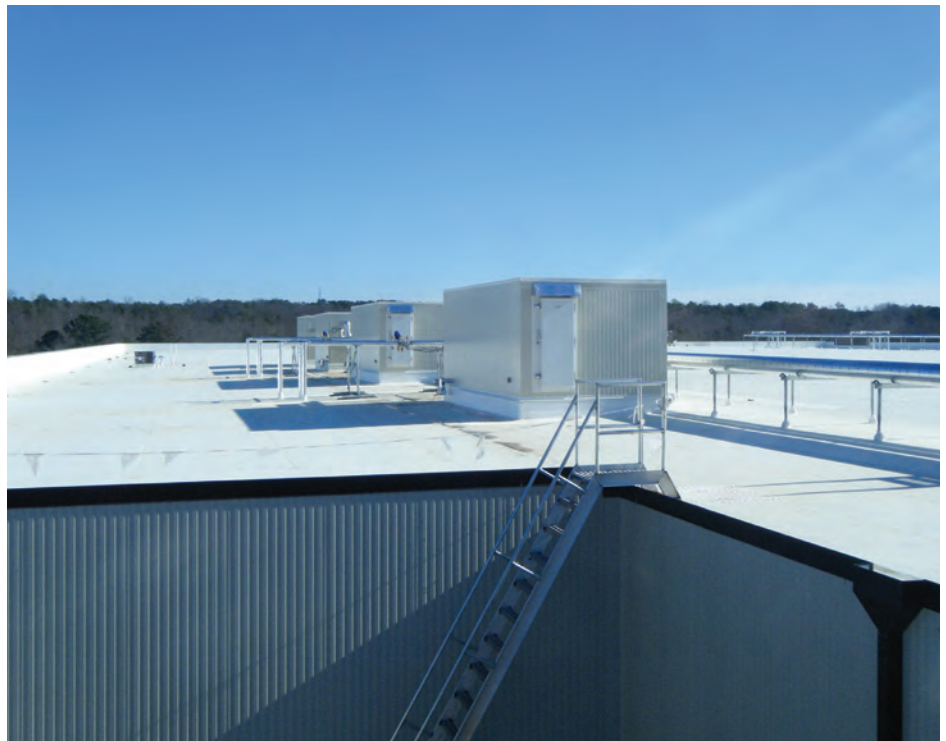
New mini-penthouses with all refrigeration and electrical complete. (Photo courtesy of ARCO Design/Build and ALTA Refrigeration.)
