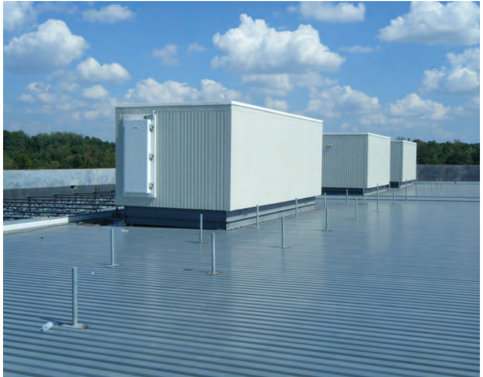
Mini-penthouses are placed on the roof prior to completion of the building – note the exposed joists and lack of roofing on building. At this point, piping and electrical is all that is needed for the units to be complete. (Photo courtesy of ARCO Design/Build and ALTA Refrigeration.)
