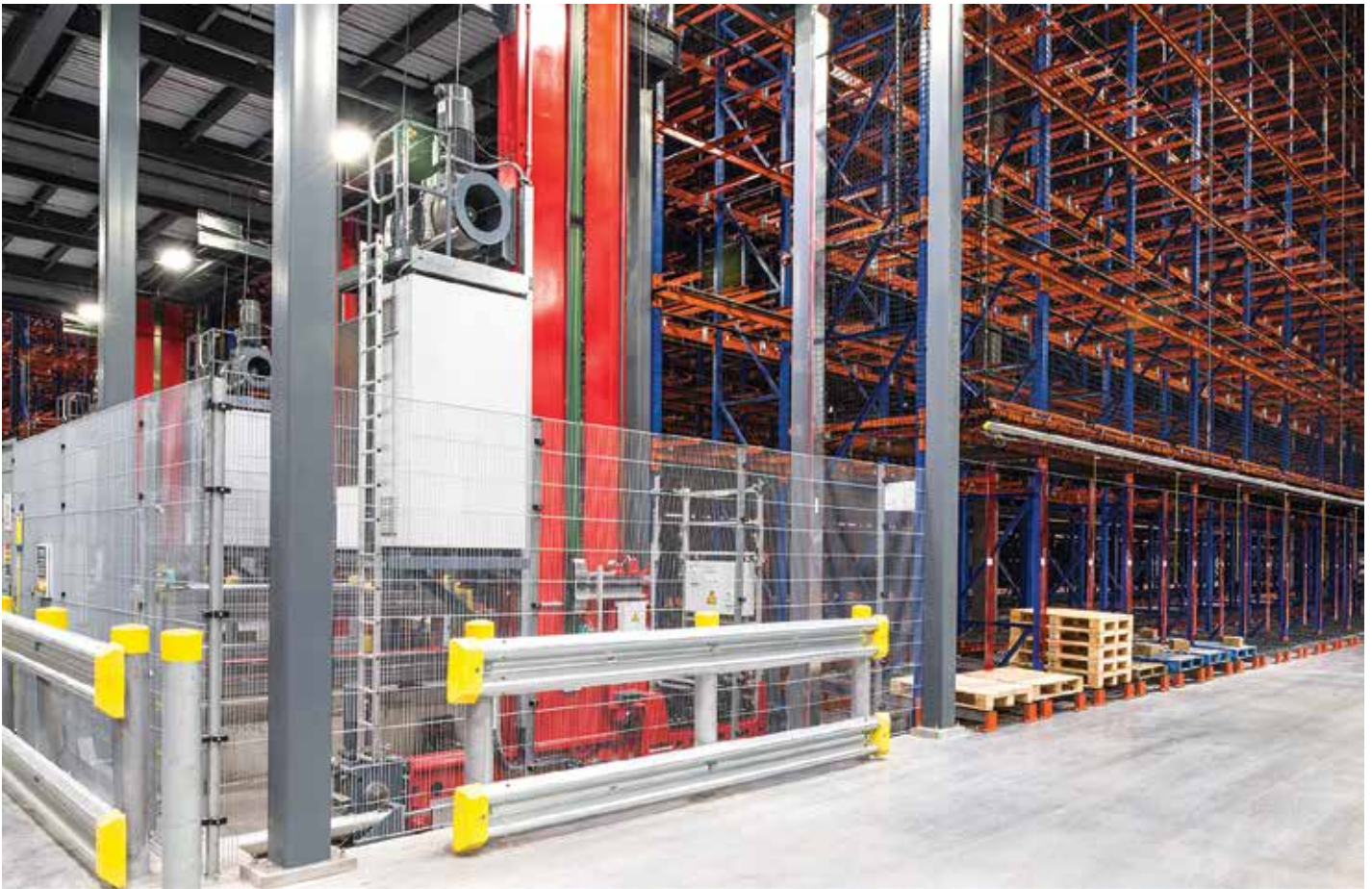
ASRS stacker crane inside an 85-foot-tall free-standing building. ASRS stacker crane stores pallets for later use and delivers pallets to pick faces for case picking order filling. (Photo courtesy of Primus Builders, Inc.)
