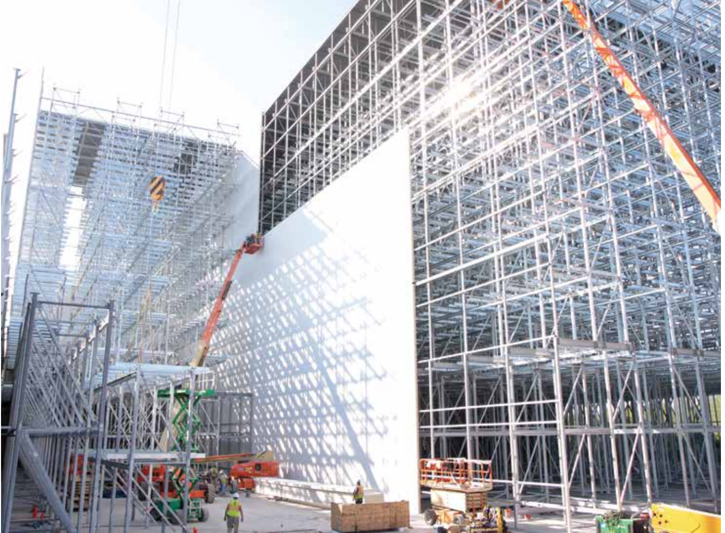
ASRS high-bay rack-supported 132-foot-tall building with ASRS stacker cranes servicing three-deep load positions and pick faces. The white wall separates the two different temperature zones in the building. (Photo courtesy of Primus Builders, Inc.)
