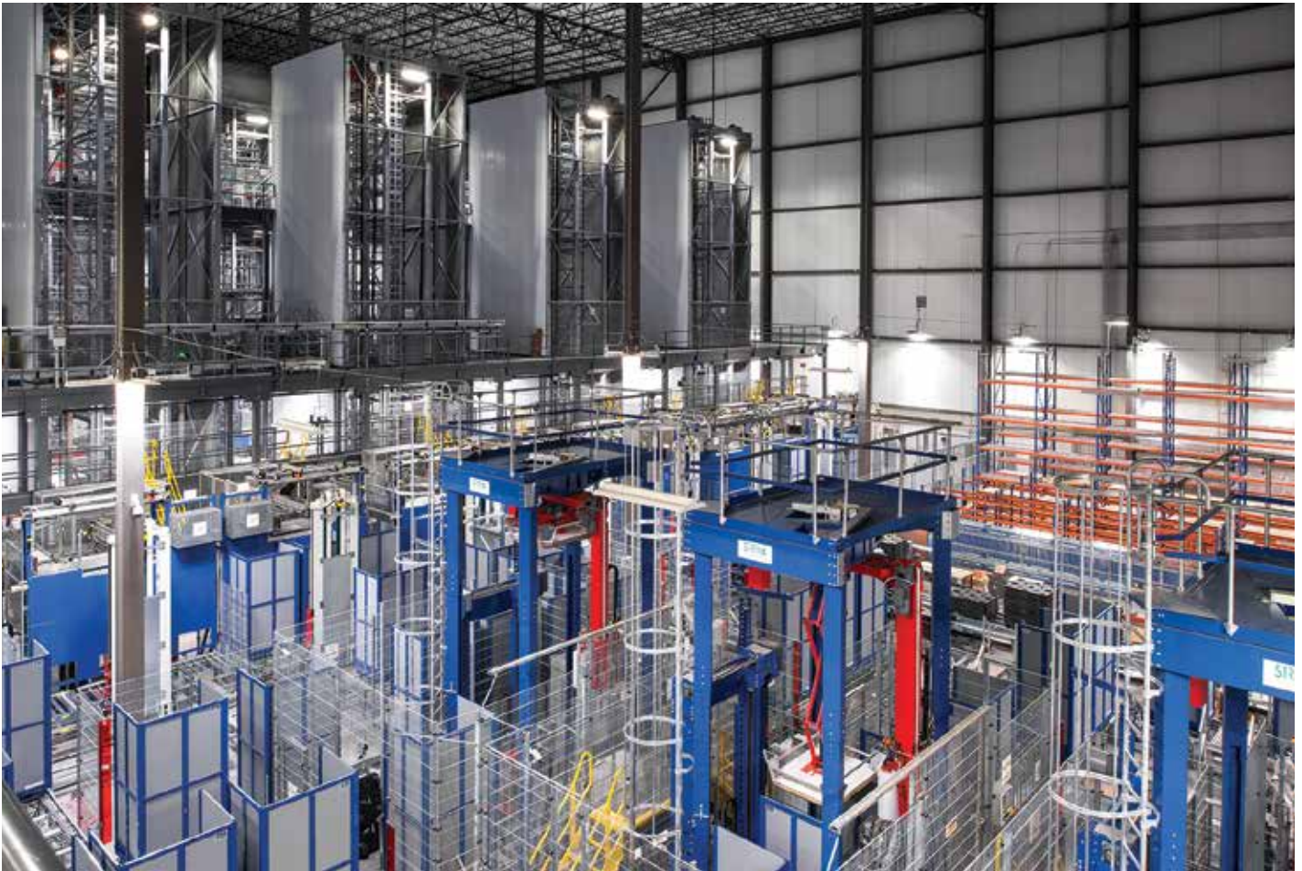
Automated order-filling area in the shipping area of ASRS facility. Shown is the robotics order filling operations for automatic case picking and order filling, stretch wrapping and shipping. (Photo courtesy of Primus Builders, Inc.)
