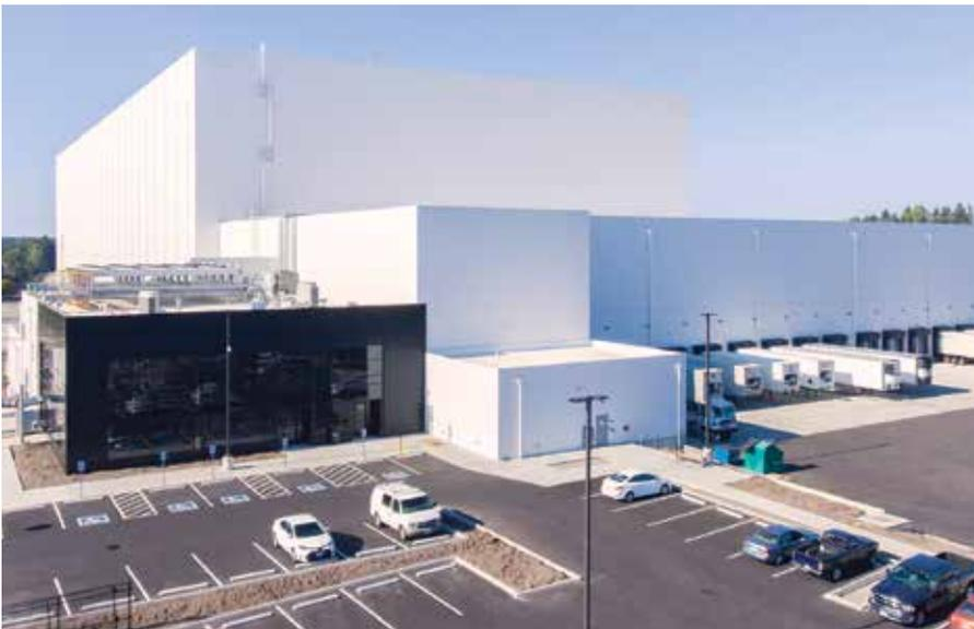
The 157,000-square-foot high-bay footprint reduces the footprint of a traditional cold storage warehouse by nearly 75 percent. (Photo courtesy of Fisher Construction Group.)
