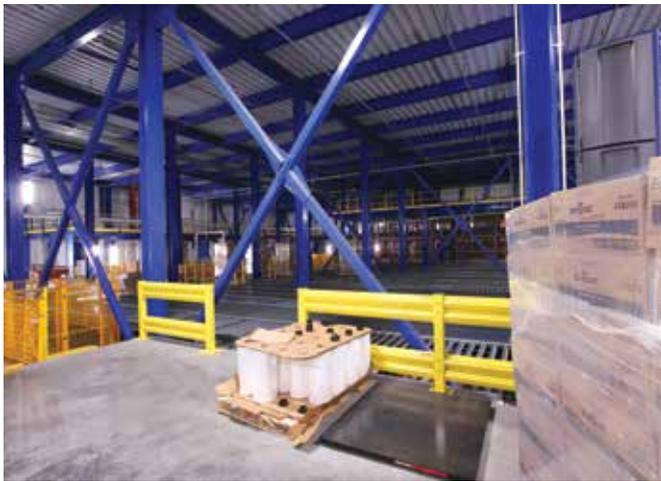
Uninterrupted pallet racking with unobstructed areas within can reach 135 feet. (Photo courtesy of Fisher Construction Group.)
