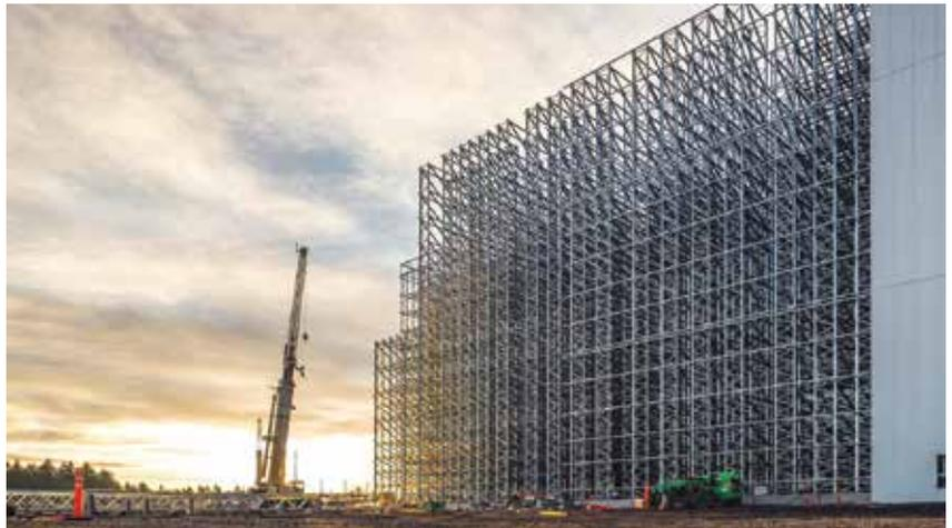
The NewCold Tacoma state-of-the-art freezer is a joint design effort by Netherlands-based NewCold Advanced Cold Logistics and the design/build firm Fisher Construction Group of Burlington, Washington. It is one of the largest cold storage facilities in the United States, with Phase 1 containing approximately 25 million cubic feet of storage capacity an 103,000 pallet positions. ((Photo courtesy of NewCold.)
