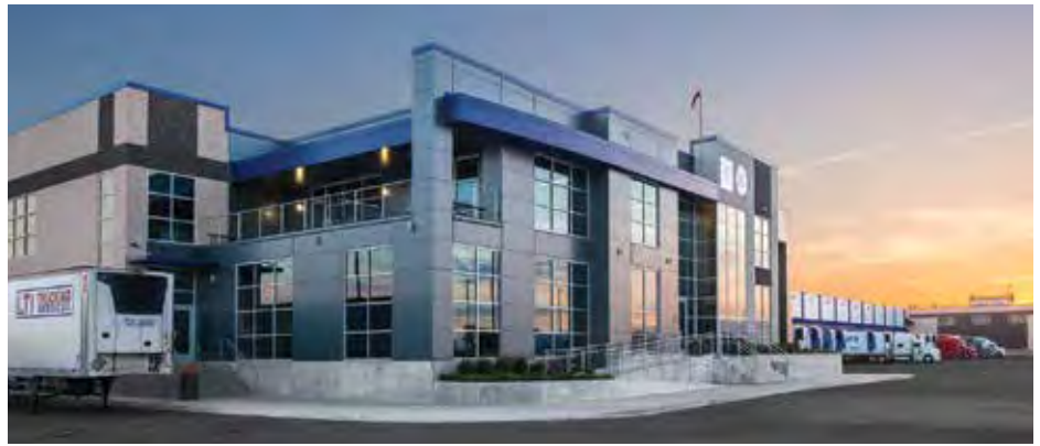
The original goal for Primus’ United States Cold Storage project in Covington, Tennessee, was LEED Silver. By closely collaborating, the team was able to identify additional LEED points that led to the project achieving LEED Gold certification. (Photo courtesy of Primus Builders.)
