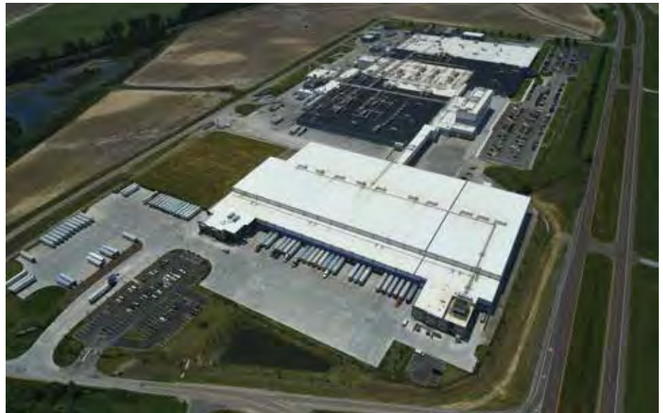
An aerial shot of the United States Cold Storage facility in Covington, Tennessee with the adjacent food processing facility in the background. (Photo courtesy of United States Cold Storage.)
