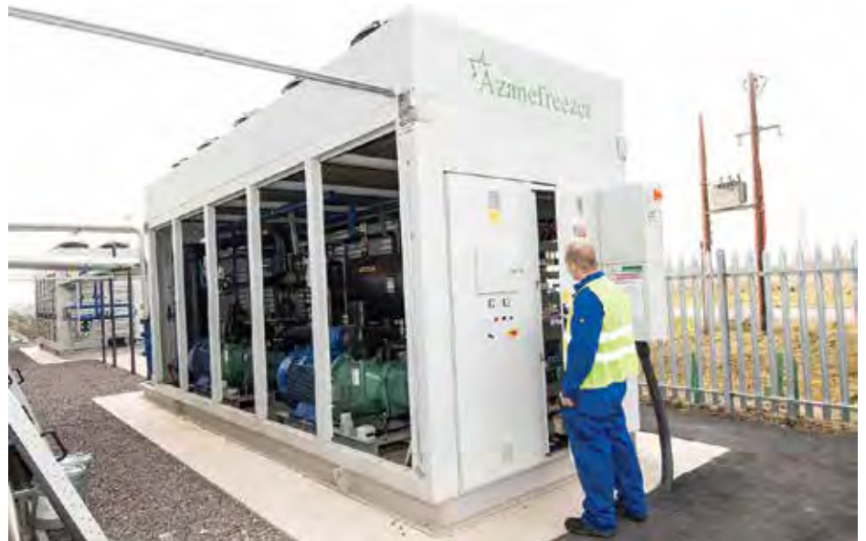
The 168 TR Azanefreezer was installed by a major frozen food distribution chain, significantly reducing energy and costs.
