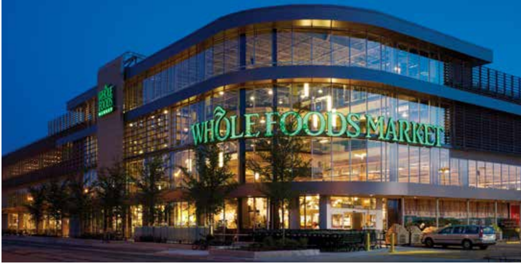
The third-largest Whole Foods store in the world, located in Lincoln park, IL, was made possible by integrating Metl-Span insulated metal panels with other metal building projects.
