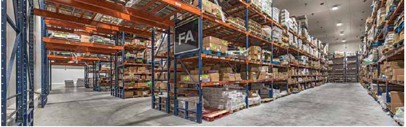
The original dry warehouse was converted to refrigerated storage and processing spaces with a system of insulated metal panel walls, liner panels, baffles and ceilings. (Photo courtesy of A M King.)
