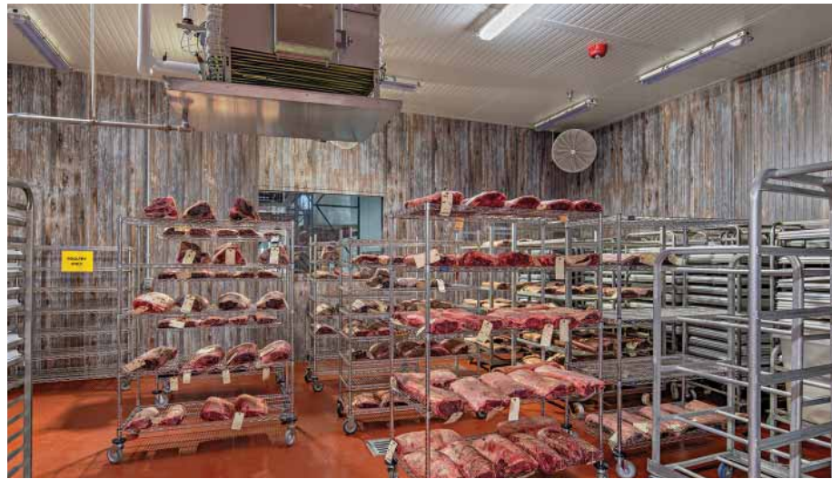
A distinctive 34-degree, 4,200-square-foot dry beef aging room is fitted with high-tech temperature and humidity controls and large viewing windows for customers. (Photo courtesy of A M King.)
