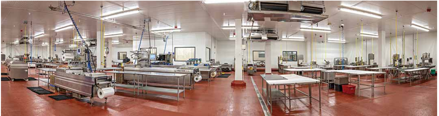
A high-strength industrial floor coating over all concrete slabs in the food processing area prevents food particles from absorbing into the concrete slab and minimizes the risk of bacterial growth. (Photo courtesy of A M King.)
