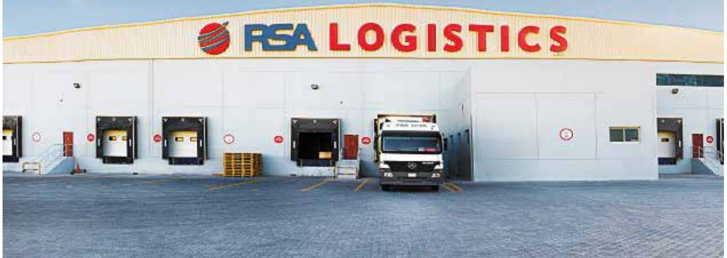
An RSA Logistics temperature-controlled warehouse facility. Warehousing in Dubai represents 16 percent of the logistics market. (Photo courtesy of RSA Logistics.)
