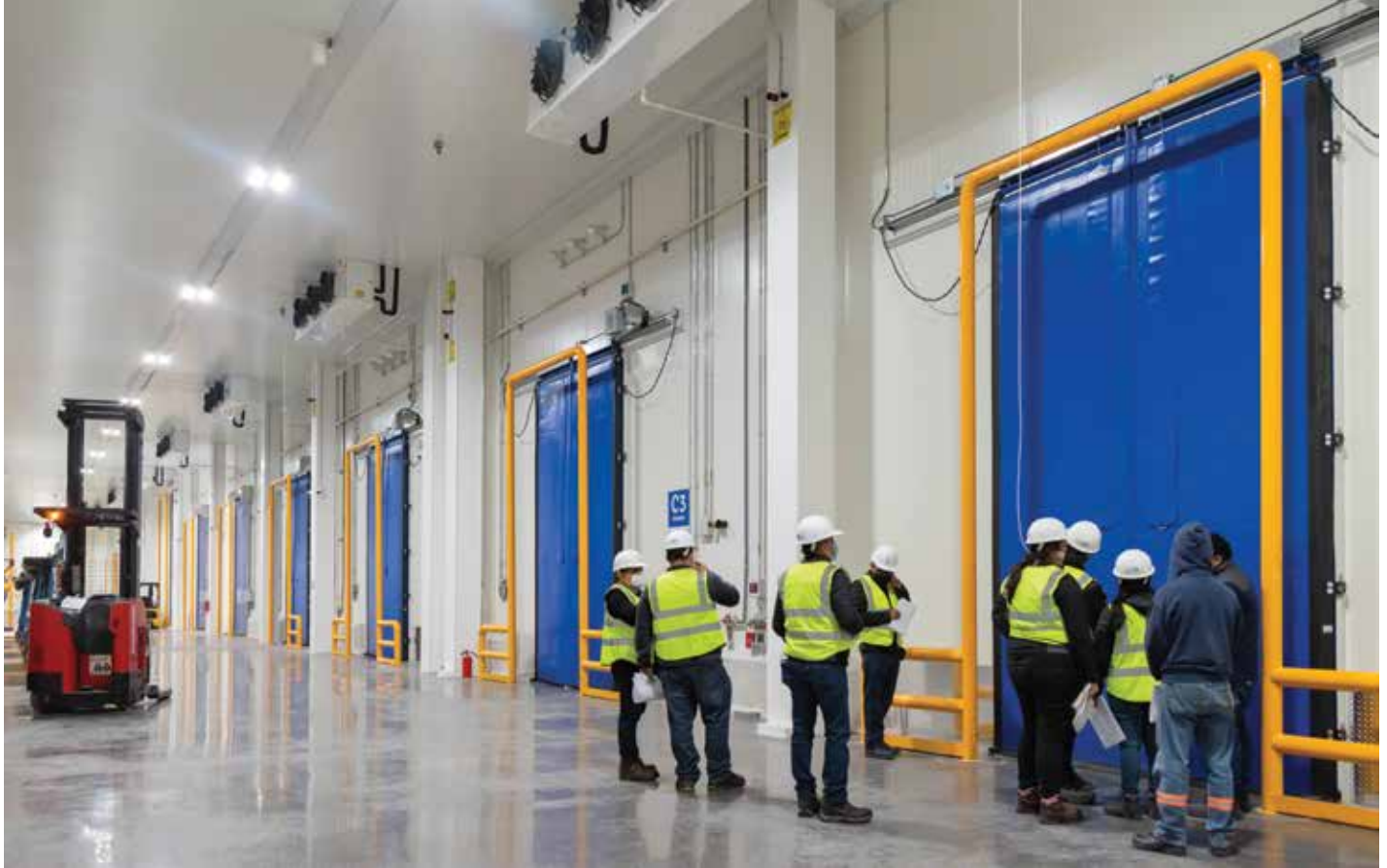
Loading dock at the new Mexideli distribution center. (Photo courtesy of SRT.)
