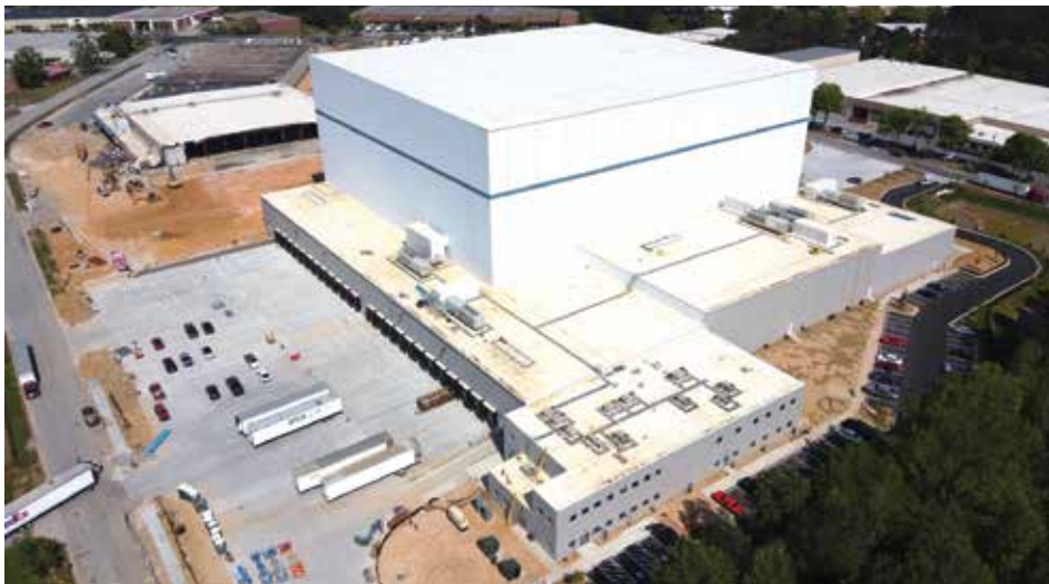
(Photo courtesy of Griffco Design/Build.)
