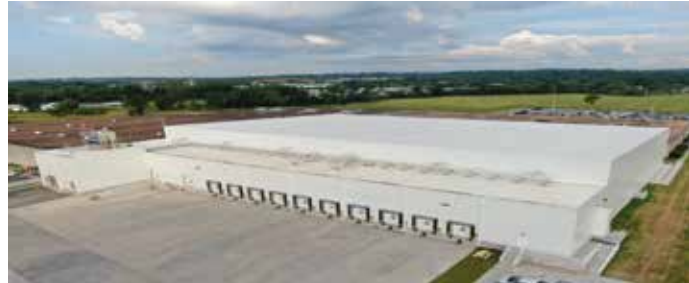
Winchester Cold Storage, Winchester, Virginia
