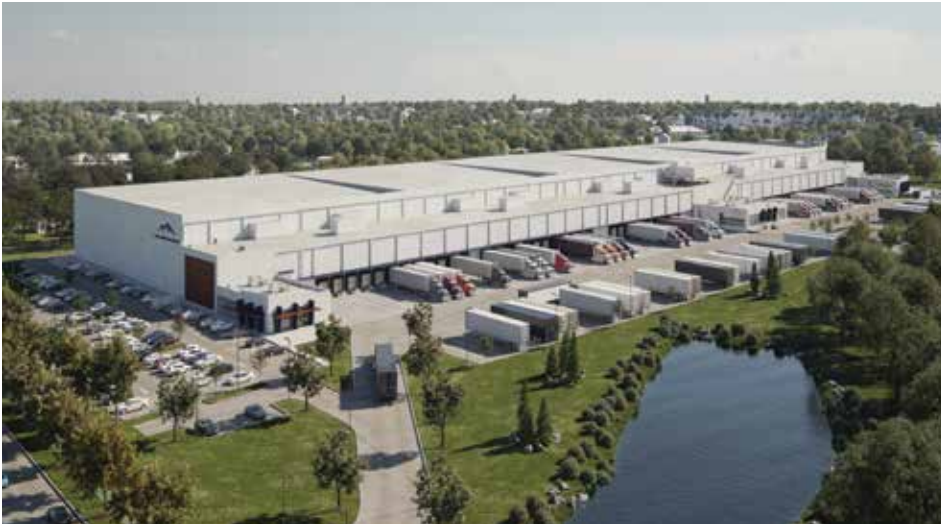
(Photo courtesy of Primus Builders, Inc.)
