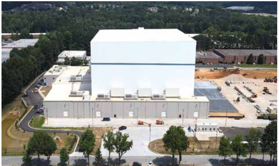
Americold Logistics’ Gateway project encompassed the demolition of a 440,000-square-foot existing cold storage building and the construction of a new, 200,000-square foot automated freezer facility. (Photo courtesy of Griffco Design/Build.)
