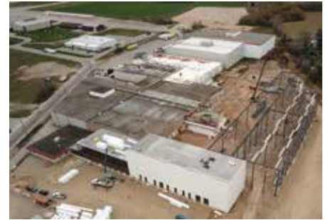
Confederation Freezers' expansion built by Coldbox. (Photo courtesy of Coldbox.)
