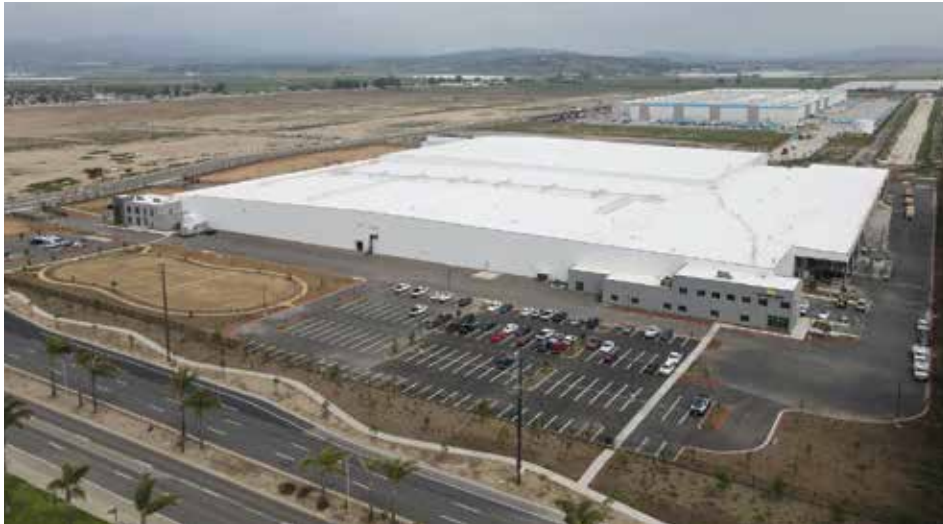
(Photo courtesy of Fisher Construction Group.)
