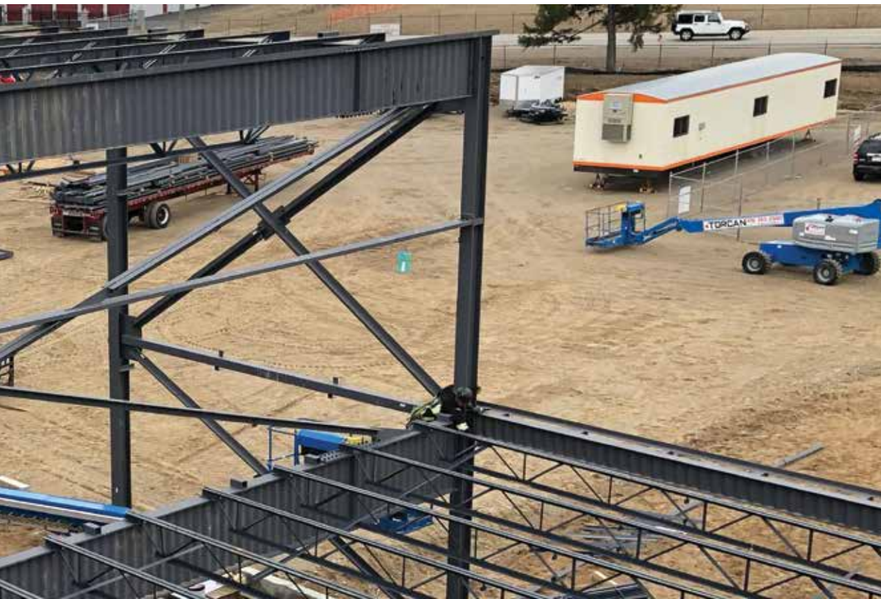
The vertical member of each SIN beam has an undulating profile allowing the structural integrity of the beam to be maintained using less steel. (Photo courtesy of Coldbox.)
