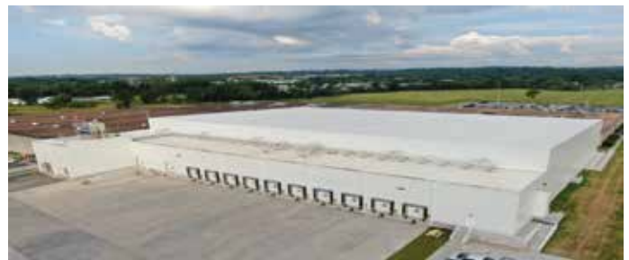
Winchester Cold Storage, Winchester, Virginia
