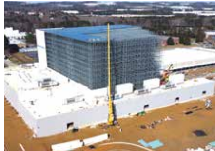
Americold Logistics' Gateway project built by Griffco Design/Build, Inc. (Photo courtesy of Griffco Design/Build.)
