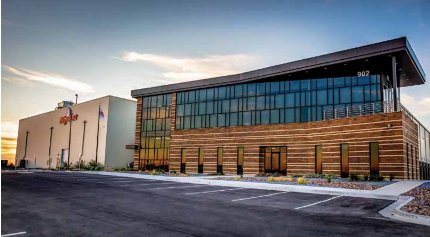
The front entry of the main office features high-performance glass. The lower level uses masonry to mitigate high temperatures during the day, low temperatures at night and reflects the natural color pallet of the surrounding landscape. (Photo courtesy of A M King.)
