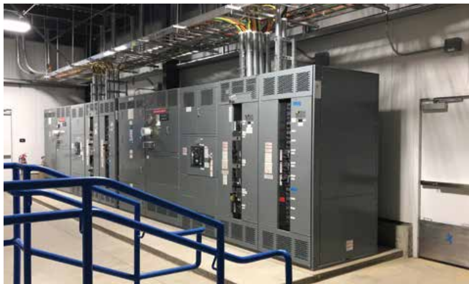
A shunt trip system was included in the refrigeration system to act as a mechanical fail-safe to shut down the system in the event the maximum power usage set by the power provider is exceeded. (Photo courtesy of Fisher Construction Group.)
