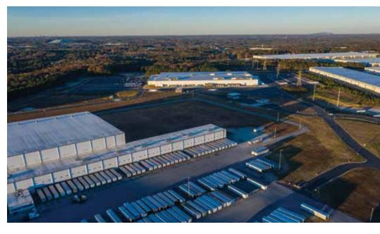
The 419,317-square-foot Kroger Fulfillment Center was designed and built by Ryan Companies U.S., Inc., has spaces for distribution, including four levels of mezzanines, office and maintenance and three temperature zones in a warehouse. (Photo courtesy of Ryan Companies U.S., Inc.)
