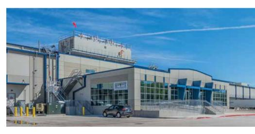
The project included a roof-top packaged refrigeration machine room, installed on the lower roof, which serves multiple tenants from one central unit but with separate utility bills. (Photo courtesy of Primus Builders.)
