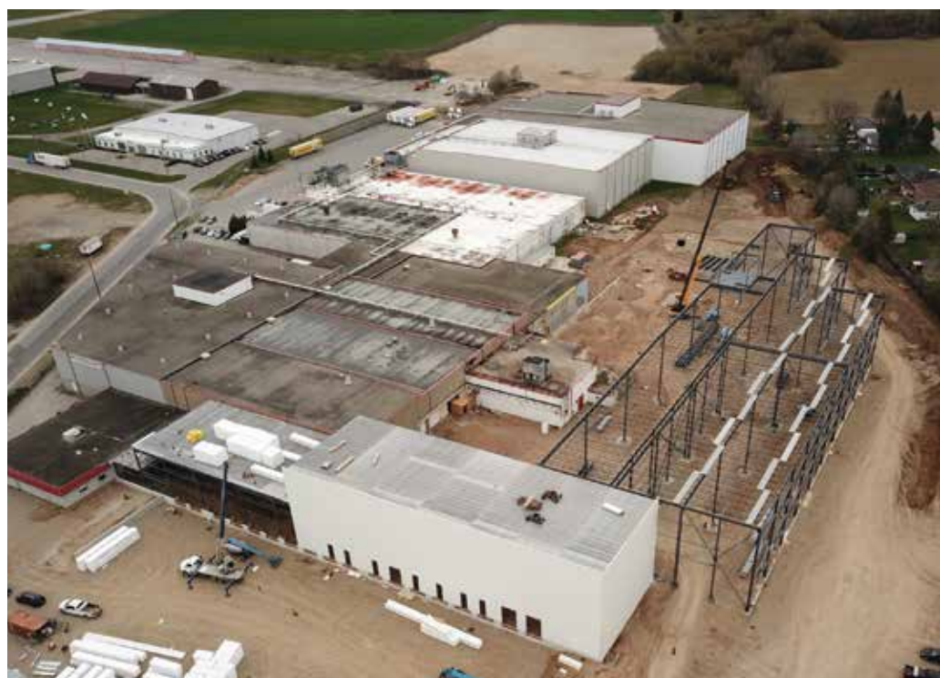
The existing facility with the new facility construction underway. The engine room is isolated (in the middle of the photo) following demolition. (Photo courtesy of Coldbox.)
