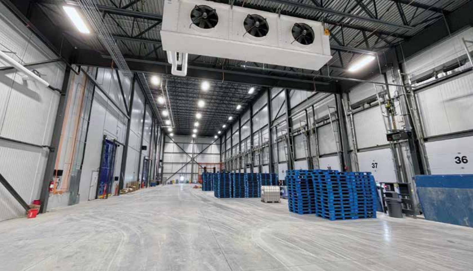
The cold dock floor system included insulation that increased the R-value, reducing the refrigeration load. (Photo courtesy of Coldbox.)
