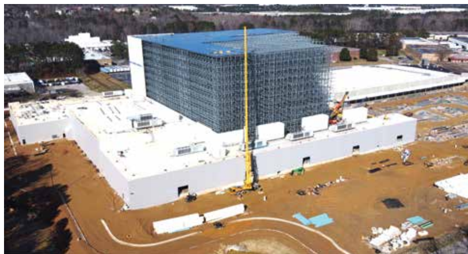
The 150-foot, -10-degree ASRS, included 41,000 pallet positions. (Photo courtesy of Griffco Design/Build.)
