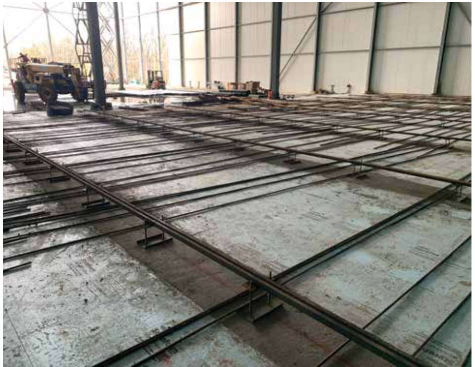
The racking rails, seen here pre-pour, had to be precision calibrated. (Photo courtesy of Ti Cold.)
