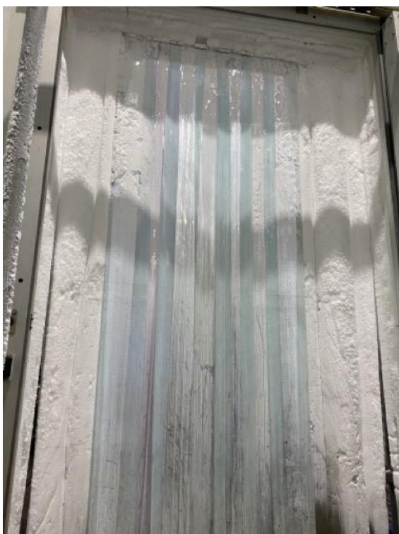
Ice build-up in doorway of frozen storage room due to open doors between room and hallway.
