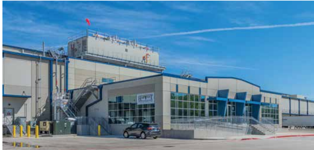
The project included a roof-top packaged refrigeration machine room, installed on the lower roof, which serves multiple tenants from one central unit but with separate utility bills. (Photo courtesy of Primus Builders.)
