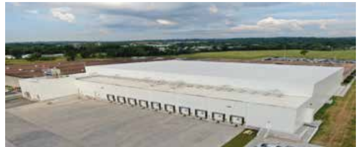
Winchester Cold Storage, Winchester, Virginia
