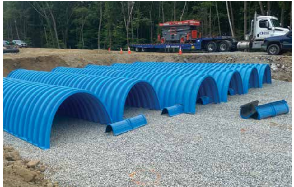
Underground storm drainage basins were used because of the tight site space. (Photo courtesy of Ti Cold.)
