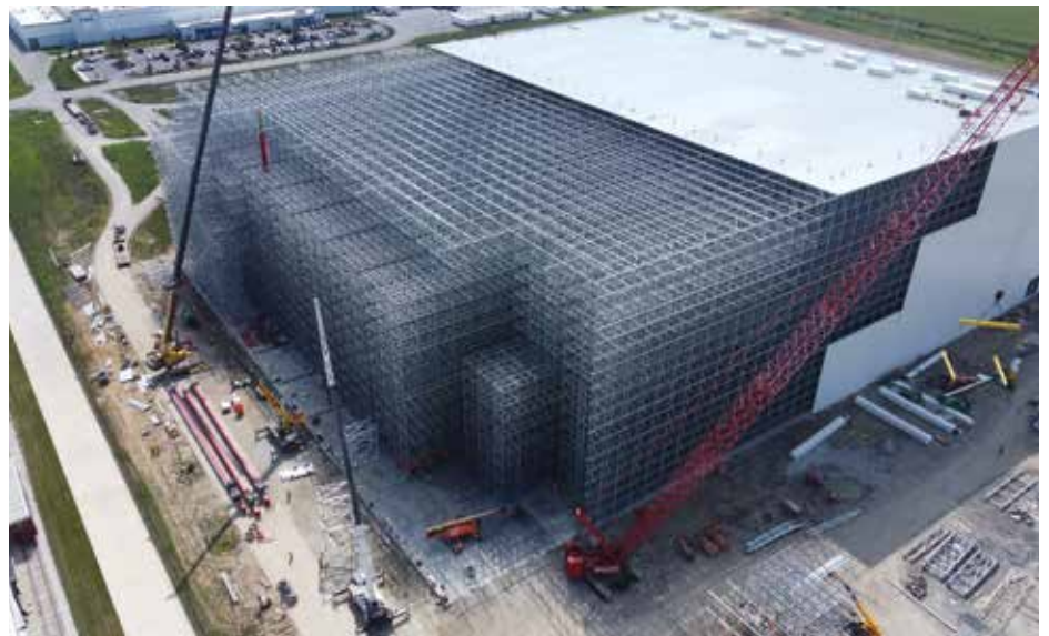
The rack-supported building, which allows for greater storage heights, is 130-feet tall. (Photo courtesy of Fisher Construction Group.)
