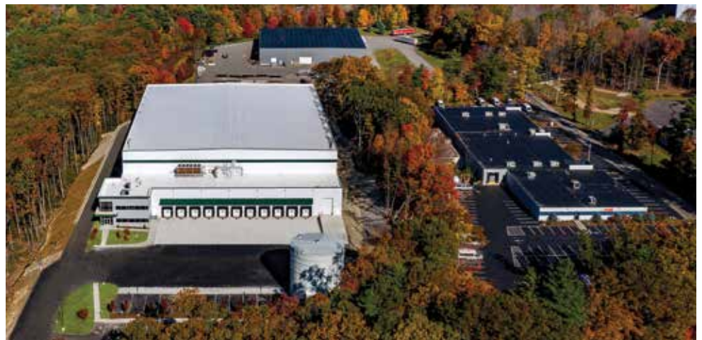
Ti Cold's 2023 Built by the Best award-winning project for Core X. The facility's tight proximity is evident in an aerial shot. (Photo courtesy of Ti Cold.)
