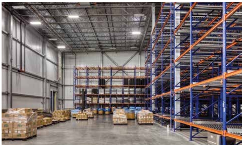
Big-D Construction designed the facility to have seven temperature zones. (Photo courtesy of Big-D Construction.)
