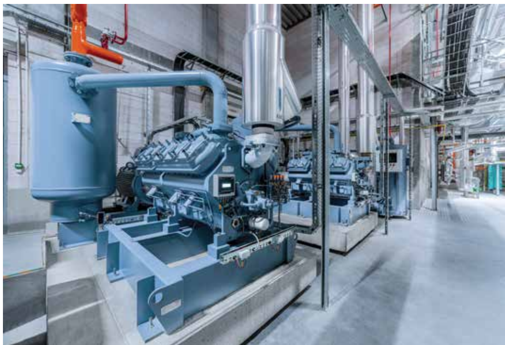
Example of GEA integrated cooling and heat pump machine room.
