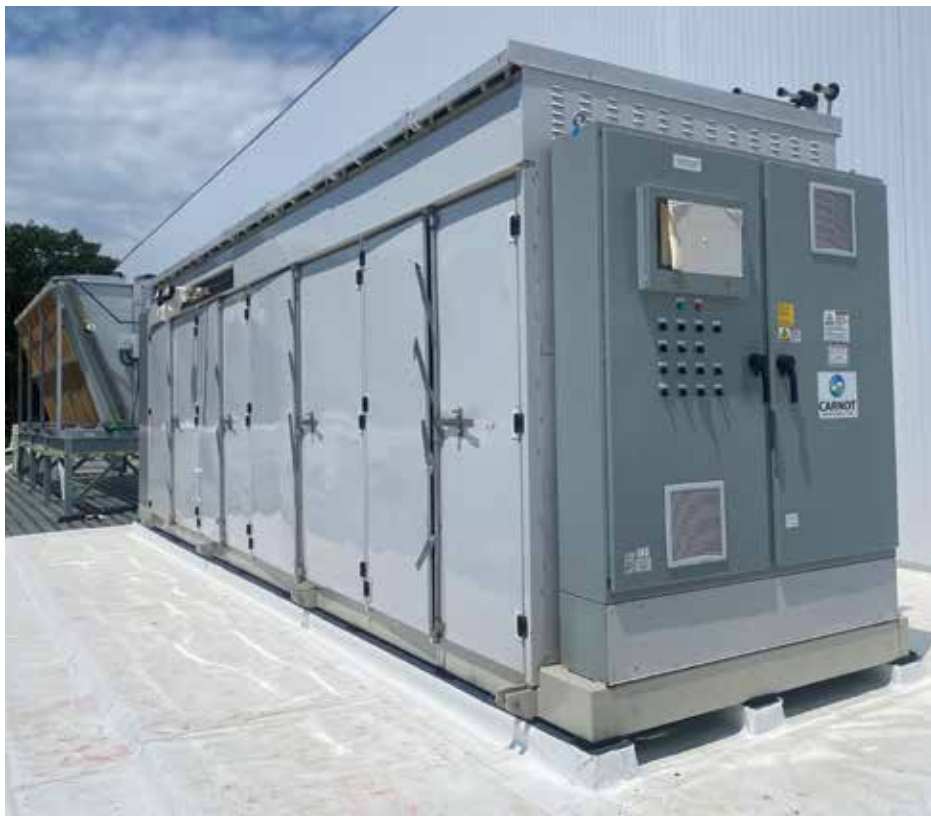
M&M Carnot's Transcritical Co2 Refrigeration System. (Photo courtesy of Ti Cold.)
