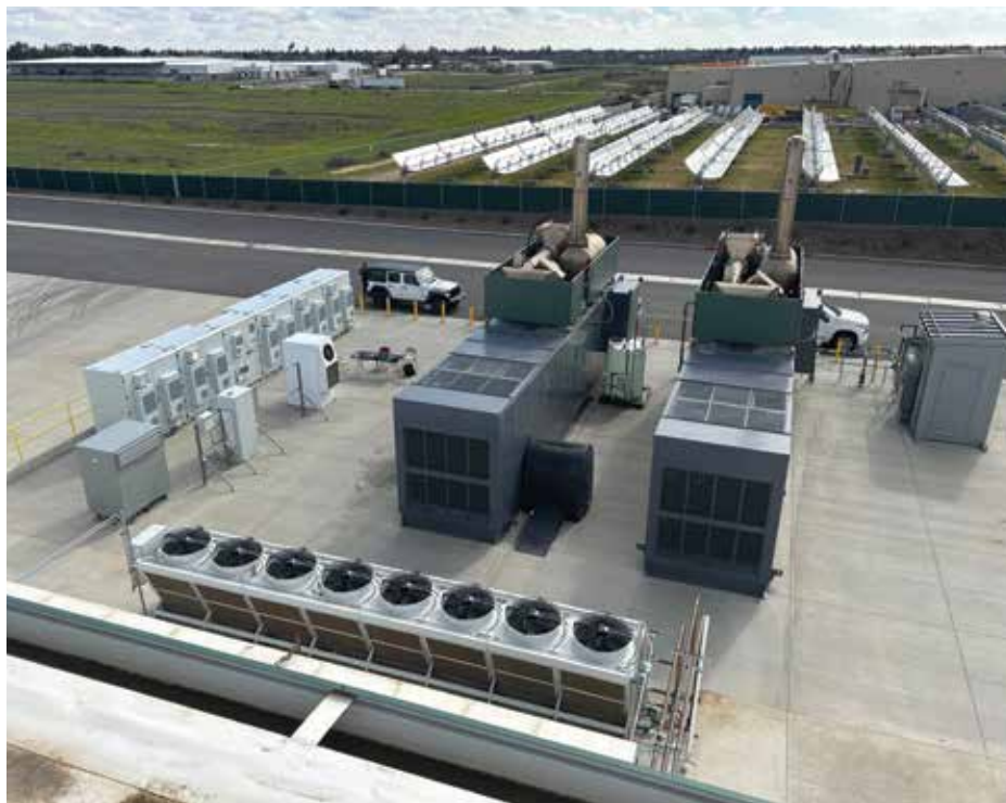
The line of white rectangular boxes to the left of the generators is a 4.8 MWh battery energy storage system. (Photo courtesy of Scale Microgrids.)
