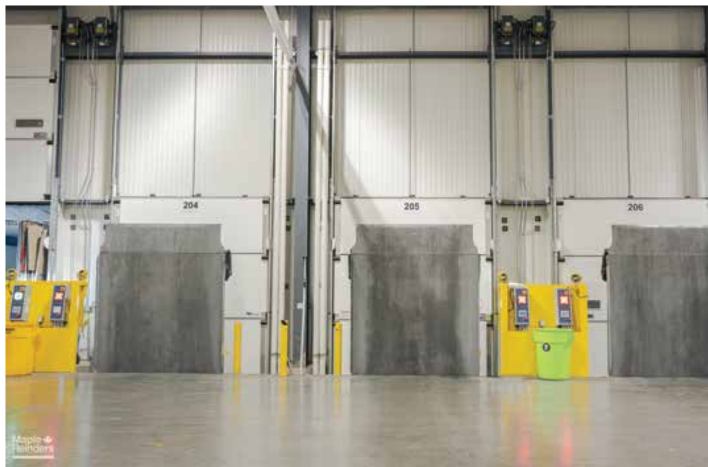
The build features a 30,000 square foot cooler/cold dock with levelers. (Photo courtesy of Maple Reinders.)
