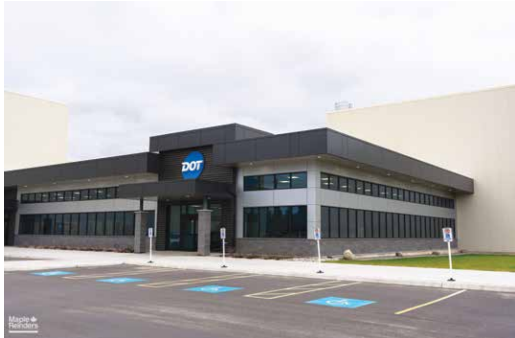
The project included 10,000 square feet of office space. (Photo courtesy of Maple Reinders.)
