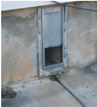
Figure 5.5 Gravity Vent Duct
