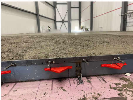
A straight, dowelled, concrete armor joint system shown as installed over XPS installation in a freezer. Courtesy Alphacon, Inc.
