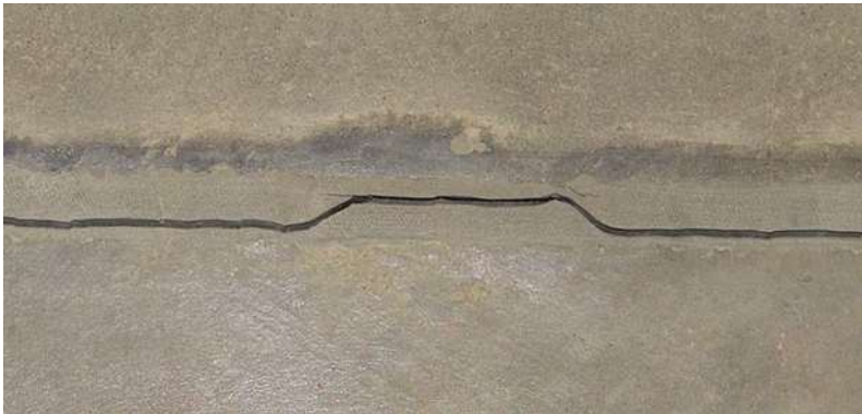
Figure 5.9 Cohesive (internal) joint filler separation
