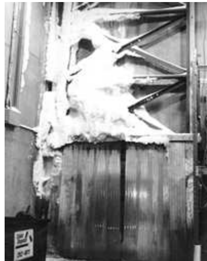
Figure 8. 2 Ice Build-up
