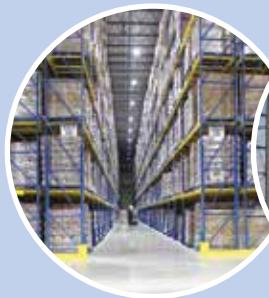
COLD STORAGE WAREHOUSING
