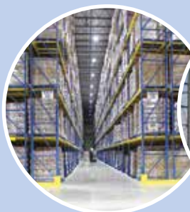
COLD STORAGE WAREHOUSING
